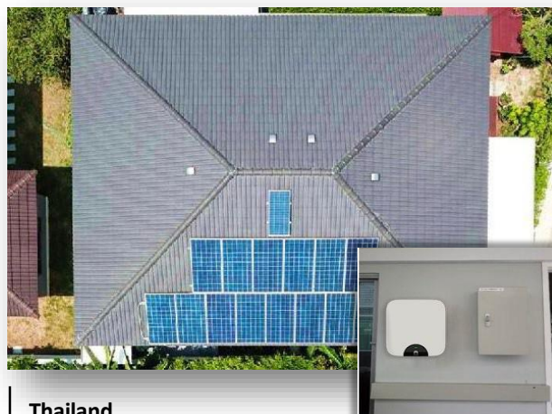
Thailand Capacity: 5kW Inverter Model: SUN2000-5KTL
