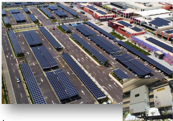
Taiwan Capacity: 4.5MW Inverter Model: SUN2000-40KTL
