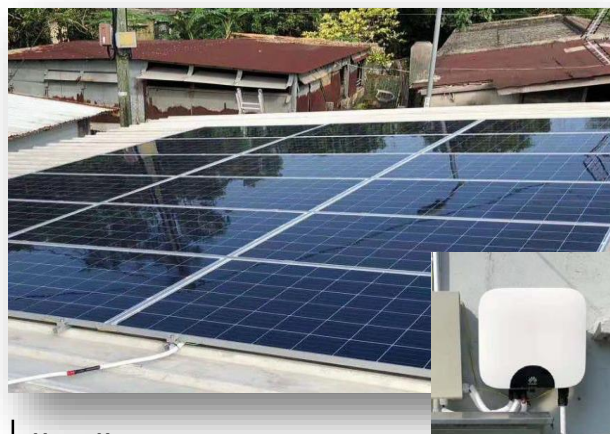
Hong Kong Capacity: 5kW Inverter Model: SUN2000-5KTL
