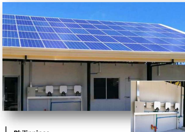
Philippines Capacity: 15kW Inverter Model: SUN2000-5KTL
