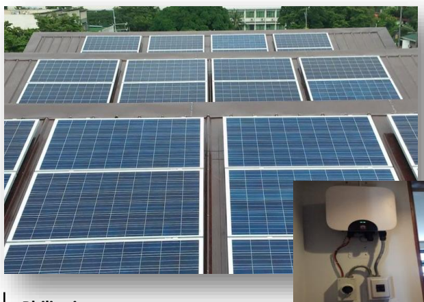
Philippines Capacity: 3kW Inverter Model: SUN2000-3KTL
